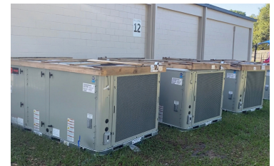
Robles Elementary School $3.6 Million - Partial A/C Overhaul, Security System, Flooring, Cooler/Freezer
