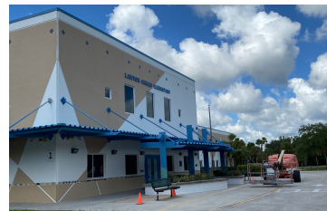
Chiles Elementary School $4.6 Million - A/C Overhaul, Flooring and Ceiling, Painting, Fire Alarm System
